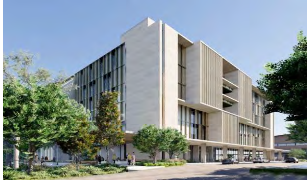
Townsville University Hospital Expansion Cost: $530m - new multi-storey clinical building
